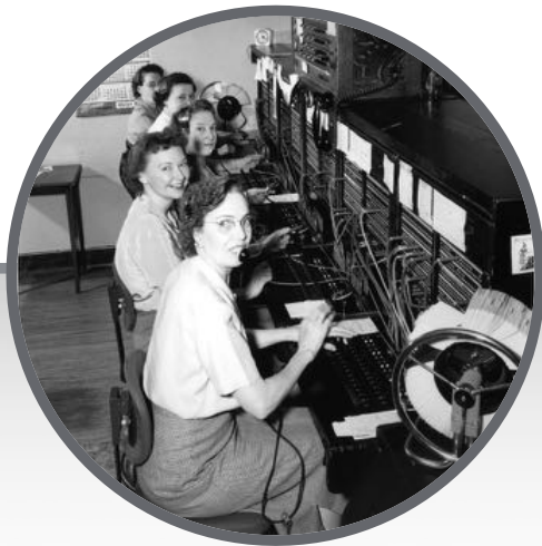
Telephone central office
